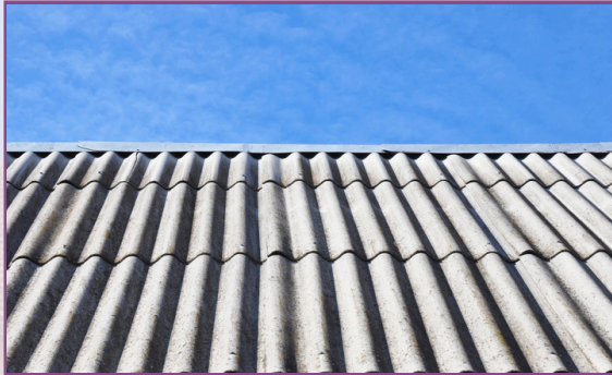
ASBESTOS ROOF TILES
