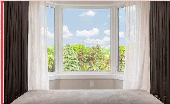
STEEL WINDOW FRAMES (PREVIOUSLY PAINTED)
