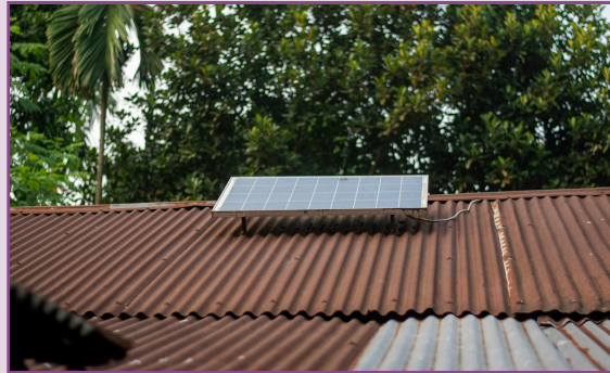
GALVANIZED METAL ROOFS
