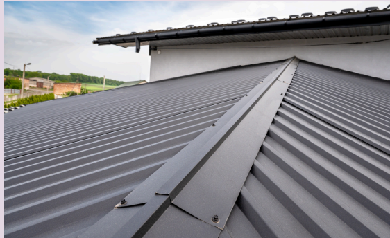
IBR METAL ROOFS
